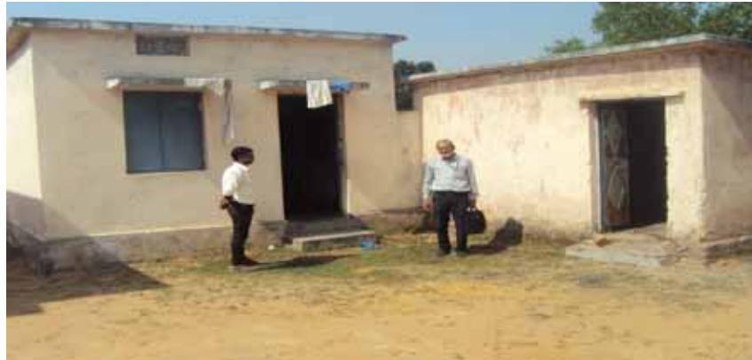
Photo 11: Multiple kitchen sheds constructed at Primary School Moliyatola, Anuppur, Madhya Pradesh dated 01 November 2014
